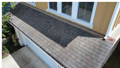
Roof Covering Material Overview
