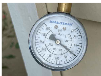
Water pressure within range
