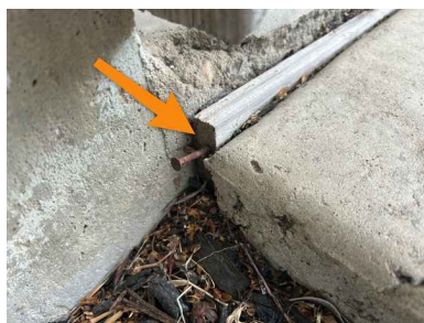
Wood to Ground Contact
