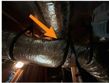
Ductwork Touching
