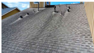
Roof Covering Material Overview
