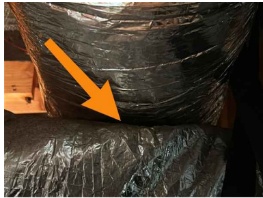
Ductwork Touching
