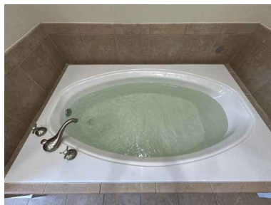
Bathtub drain/leak tested
