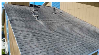
Roof Covering Material Overview
