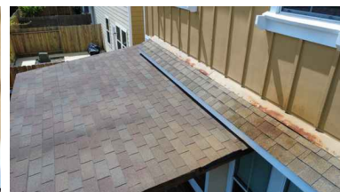
Roof Covering Material Overview
