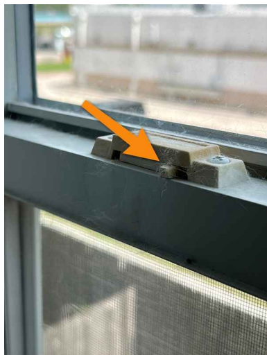
Damaged Lock
