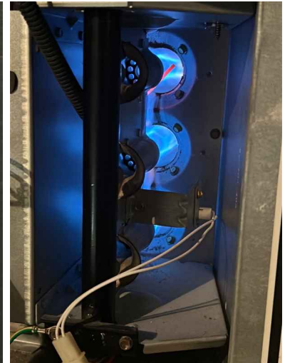
Furnace burners in operation
