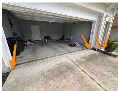
Wood to Ground Contact
