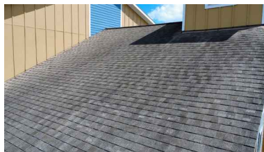
Roof Covering Material Overview
