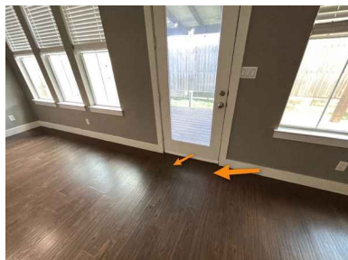
Flooring-Moisture Damaged
