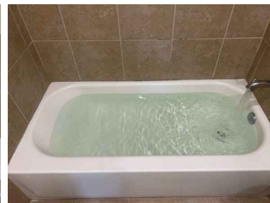
Bathtub drain/leak tested
