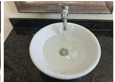
Sinks leak/drain tested
