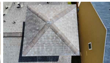
Roof Covering Material Overview
